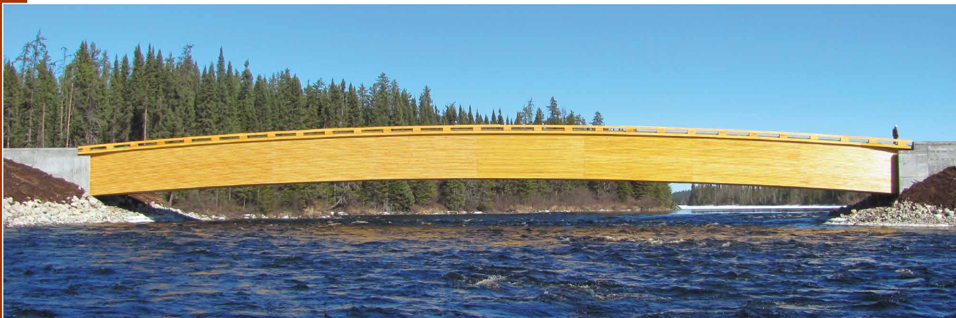
Pont Maicasagi. Photo : Nordic Structures
